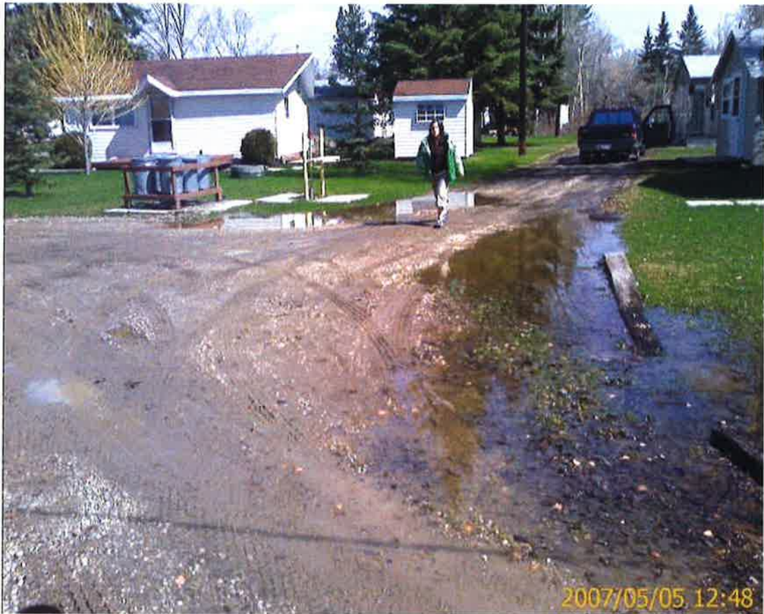
Figure 1: This photo, taken after several days of constant rain at Sunset Point Camp, illustrates close to the ideal practice for green camp water management. Gravel roads (and paths) with a good crown provide a relatively dry and permeable travel surface while forcing the water to pond near the grass. This water helps keep the site green and the fire hazard low. Infiltration and evaporation can dry the site surface in one sunny day. The camp is pleasant and useable. Maintenance requires occasional reshaping or addition of gravel to keep roads and paths dry.
