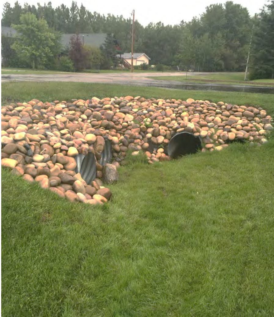
Photo 15 – F03 and F04 culvert inlet (left) and F05/F06 culvert outlet (right), facing east.
