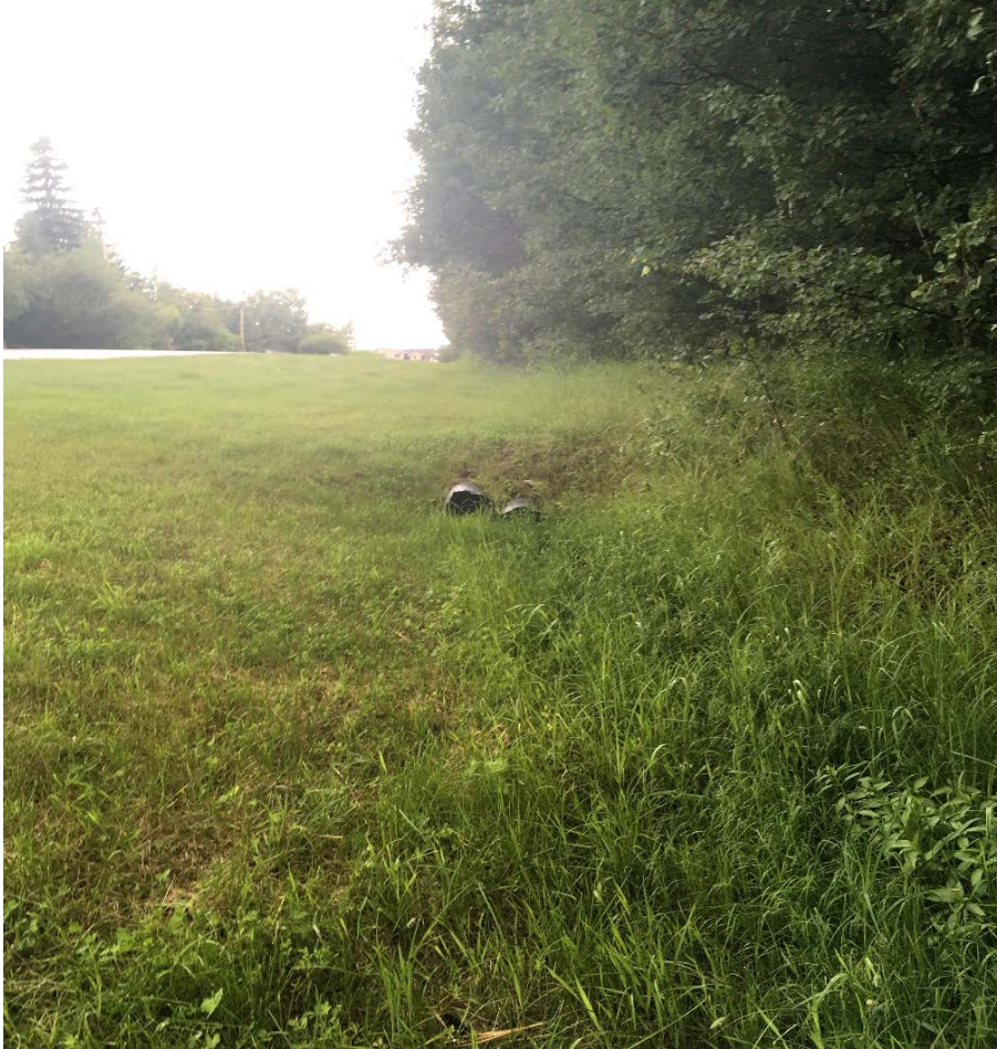
Photo 31 – Culvert I03/I02 inlet, facing west.
