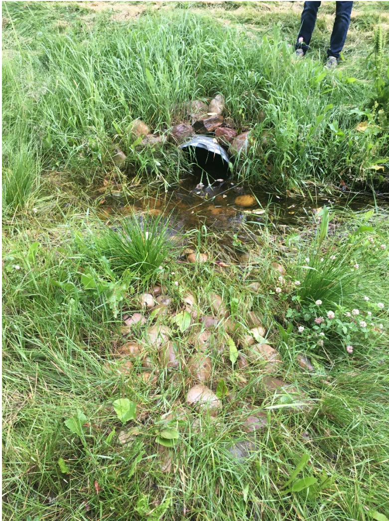
Photo 3 – Culvert RE02 outlet, facing east.
