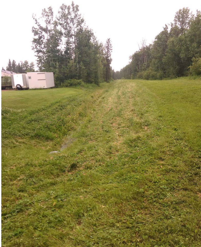
Photo 1 – Railway embankment west ditch, culvert D08 inlet, facing north.
