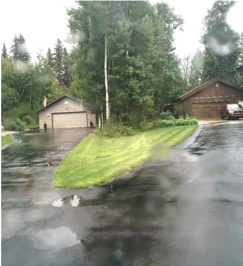
Photo 13 – 48 Street property line swale, facing east.
