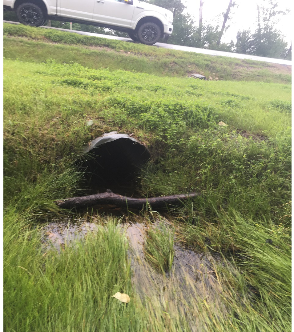
Photo 24 – Culvert F02 inlet, facing northwest.
