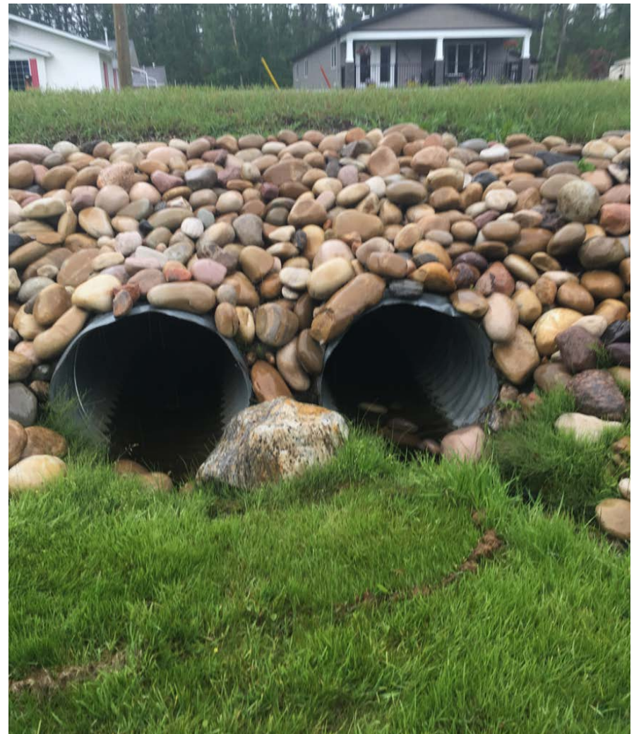
Photo 16 – F03 and F04 culvert inlet (facing north).
