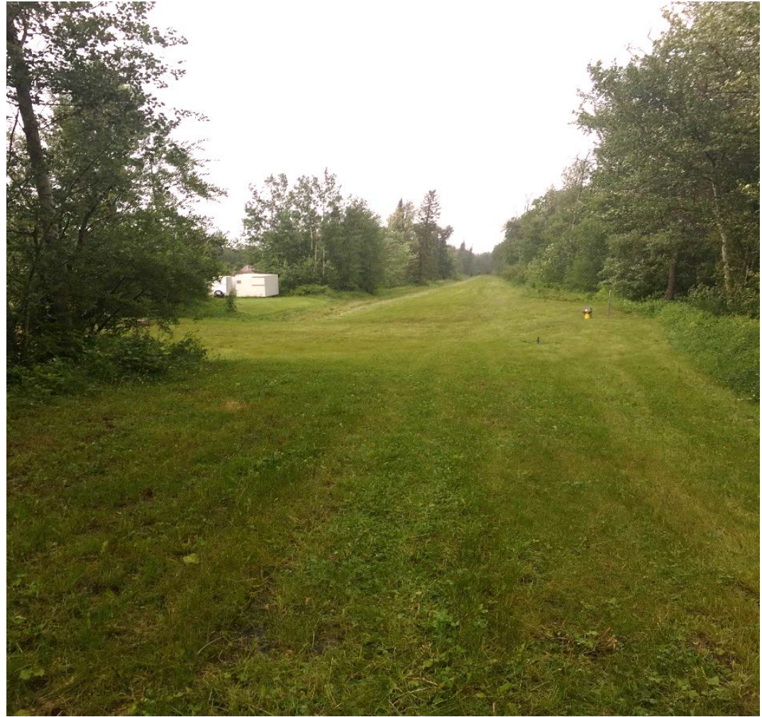
Photo 8 – Existing railway embankment recreational trail, facing north.
