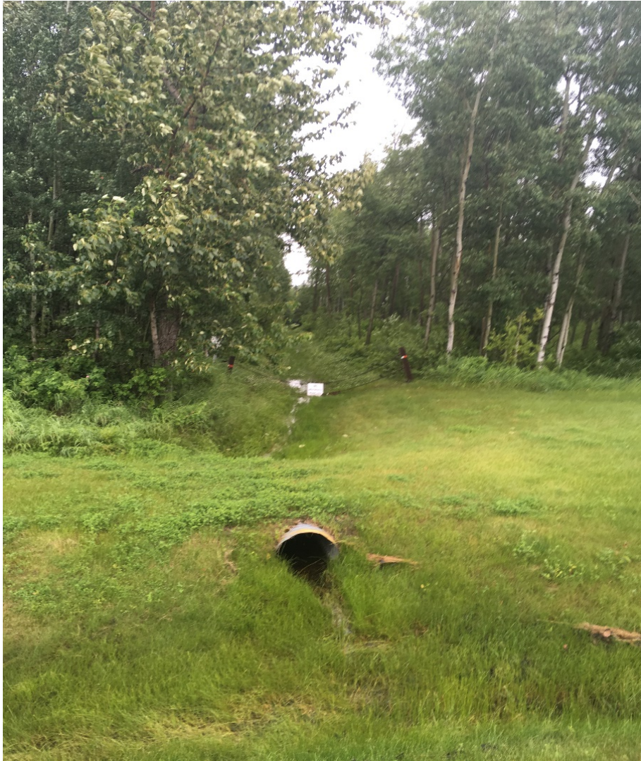
Photo 23 – Culvert F02 outlet (Sunset Drive Recreational Trail Crossing), facing east.
