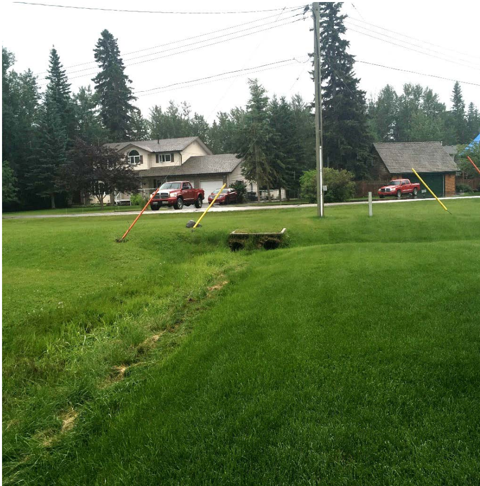
Photo 17 – Lot 7/8 swale and culvert F03 and F04 outlet, facing south.
