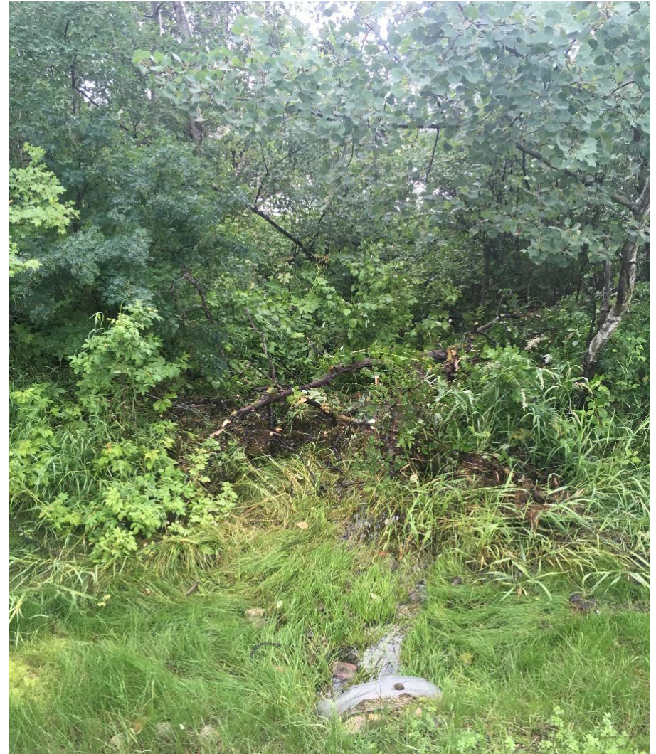
Photo 26 – Culvert F01 outlet, facing west.
