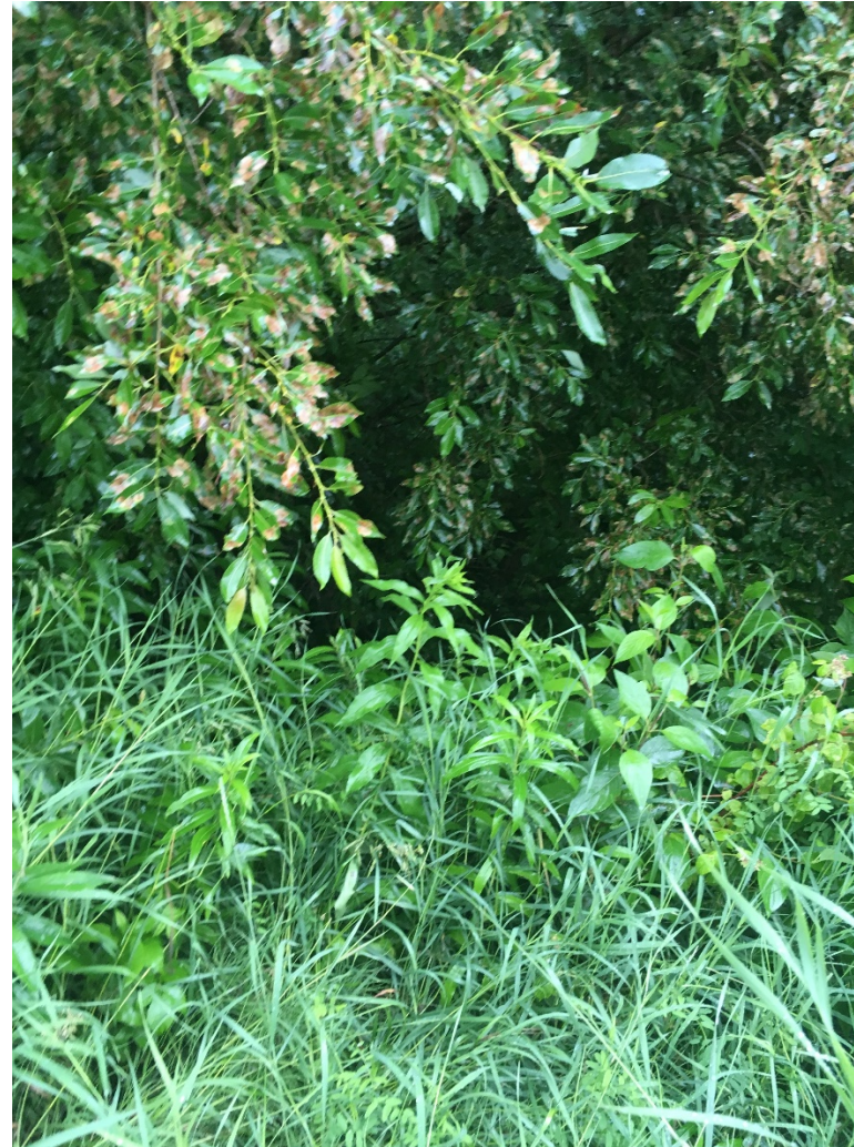
Photo 4 – Culvert RE02 inlet, facing east.
