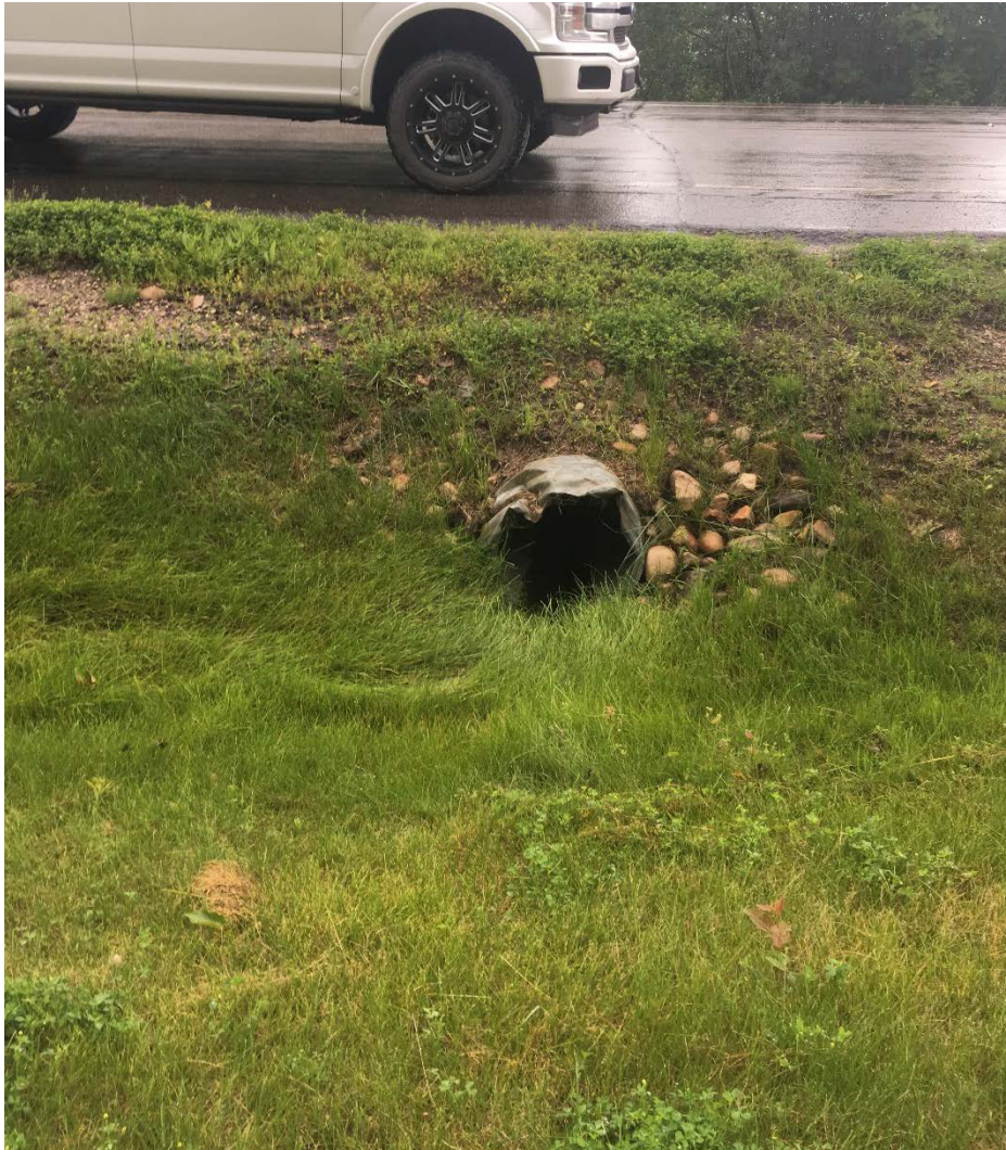
Photo 25 – Culvert F01 inlet, facing west.
