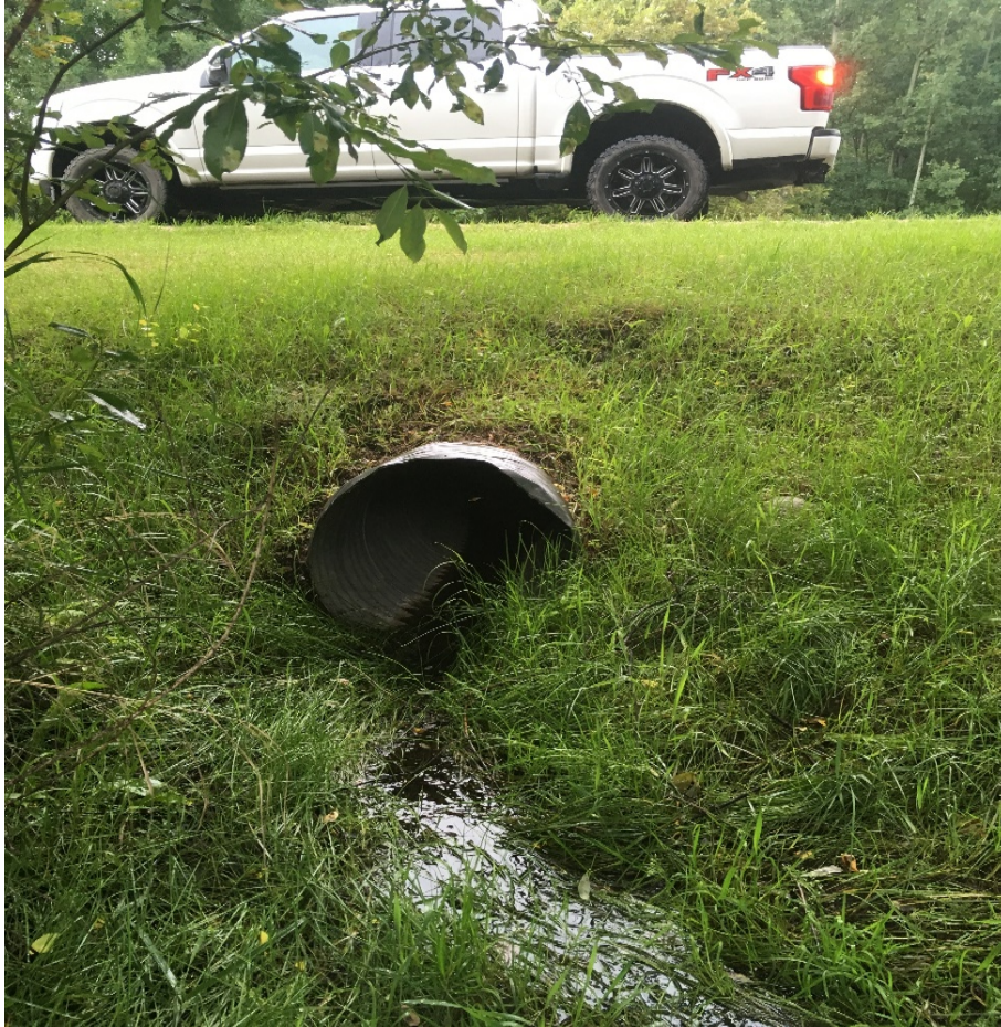
Photo 29 – Culvert I04 inlet, facing north
