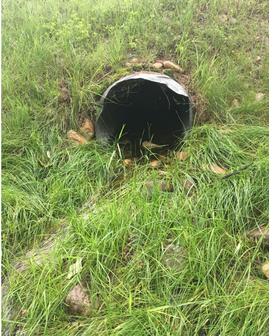
Photo 27 – Culvert F01 outlet, facing east.
