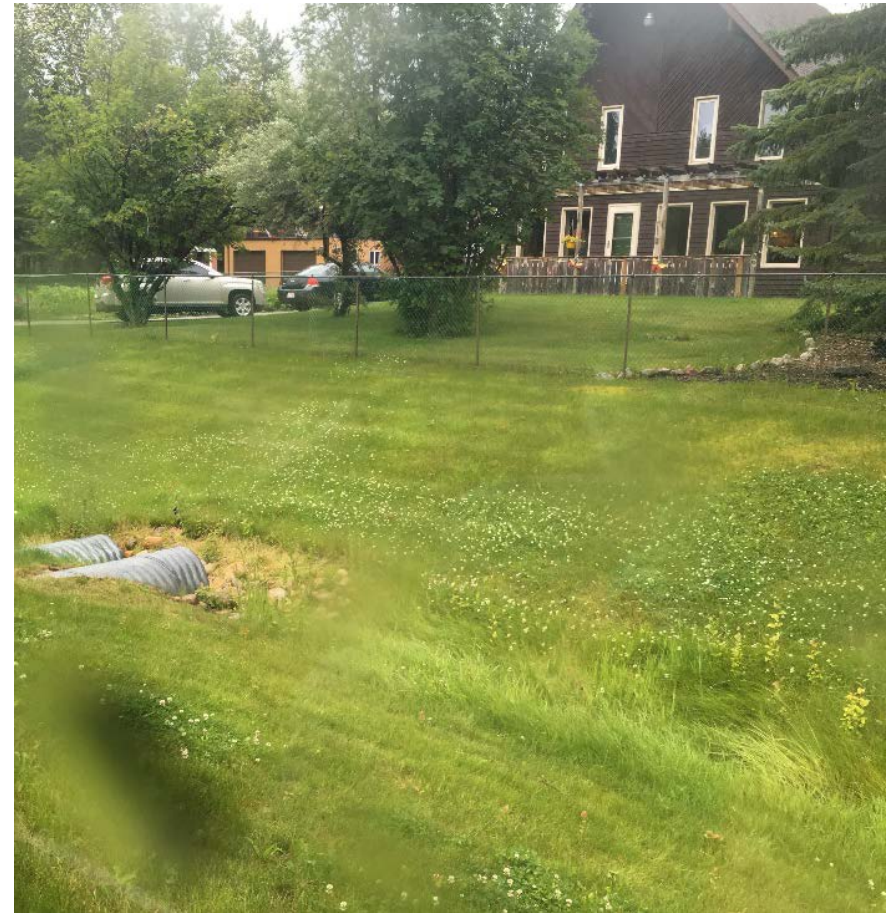
Photo 14 – Culvert F11 and F12 48 Street crossing inlet, facing east.
